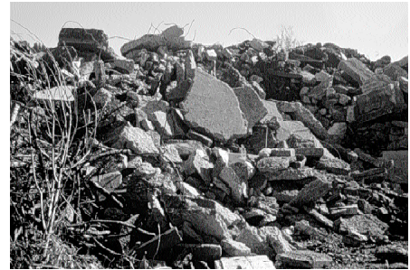
Figure 13: Concrete with rebar can be crushed and separated for recycling
