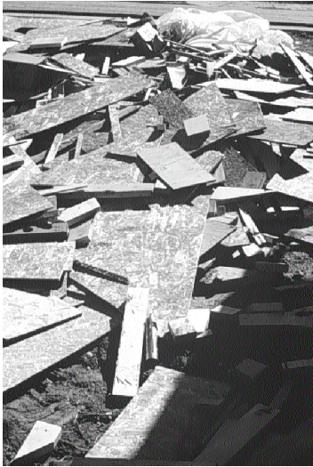
Figure 15: Time-based hauling makes sense when construction phases generate mounds of homogeneous material
