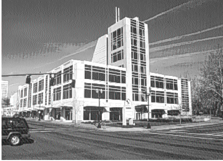
Figure 23: Metro Headquarters by Thompson Vaivoda Architects in Portland reused an existing concrete frame. (Erik Barr)
