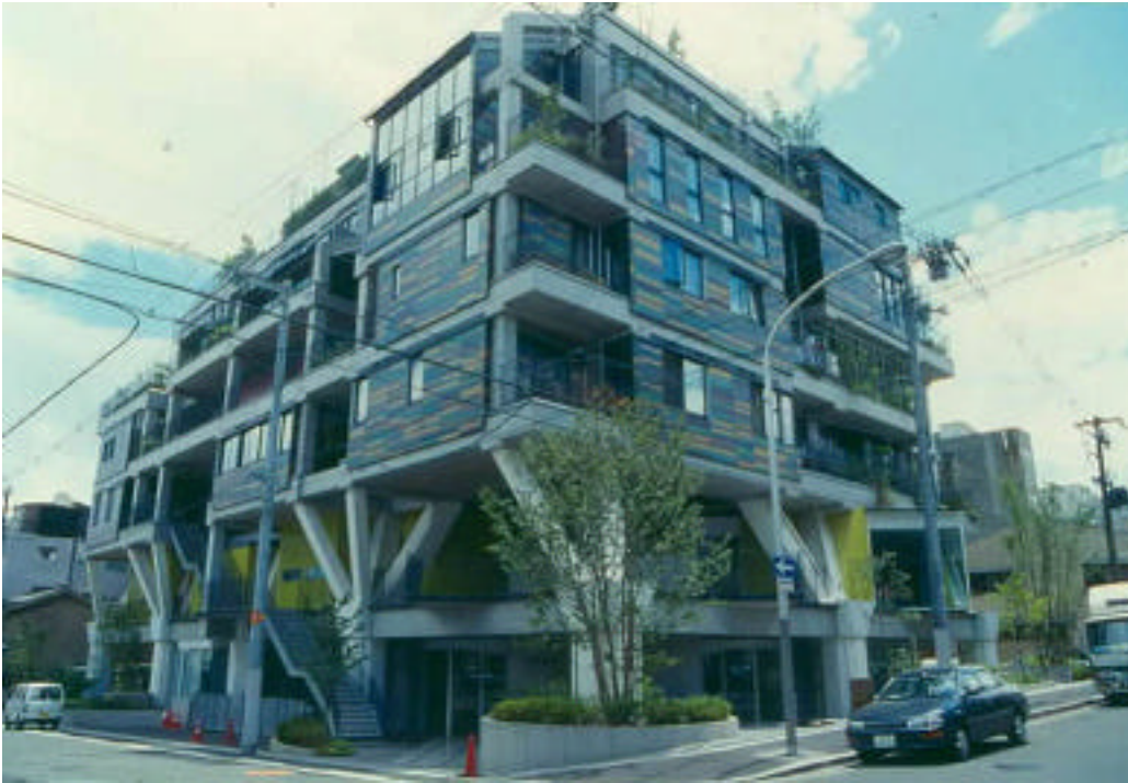
Figure 1. View from Main Access Road
