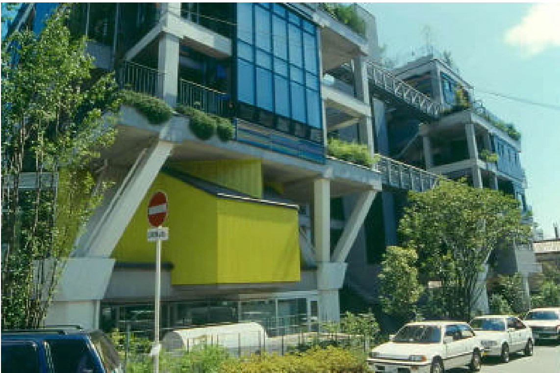
Figure 5. Branching of Support Columns
