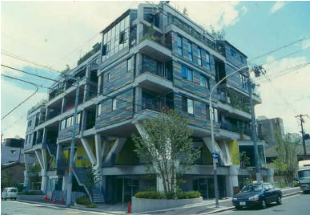
Figure 1. View from Main Access Road
