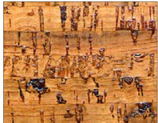
2004 05 04_Gallery Floor Replacement_7_wood
