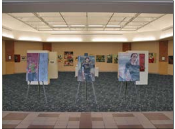
2004 05 04_Gallery Floor Replacement_rubber4
