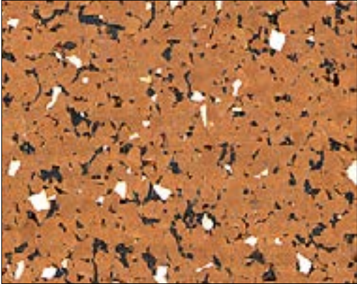
2004 05 04_Gallery Floor Replacement_4
