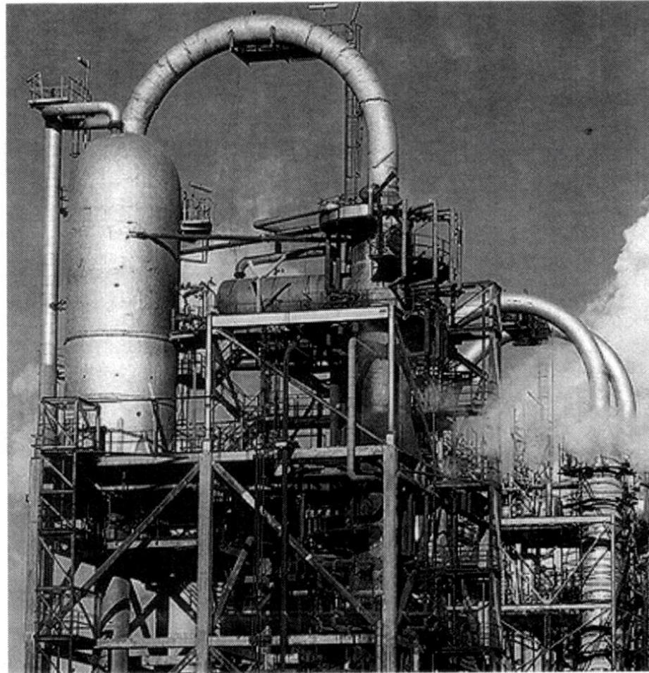
The reactor is 3.5 m in diameter and 38 m tall.
