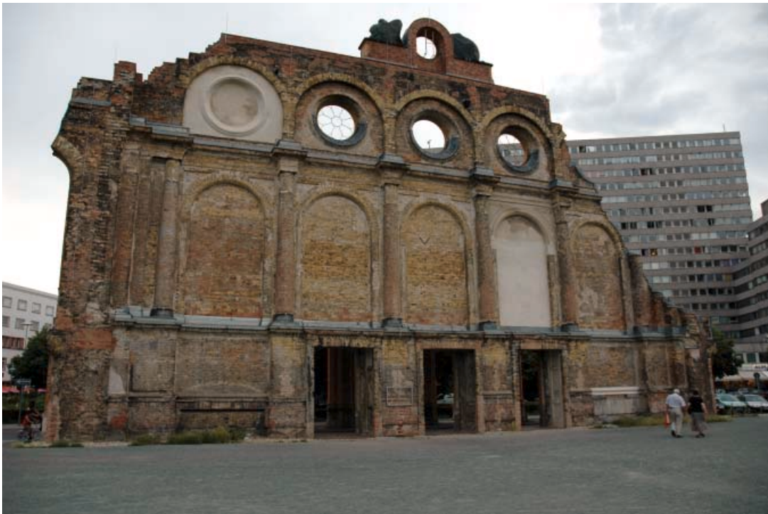
FIGURE 4. Façade of the Anhalter Bahnhof, Berlin, showing patching. Photograph by the author, June 2007.
