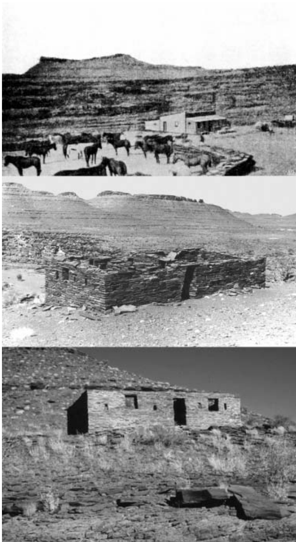
FIGURES 14–16. Top: station at Naiams, original condition (source: Grosser Generalstab 1907, 113); middle: ruins of the Naiams station before 1967 (reprinted courtesy of National Archives of Namibia, photograph no. 2635); bottom: partially restored ruins of the Naiams station, present condition (photograph courtesy of Dr Andreas Vogt, Windhoek/Namibia).
