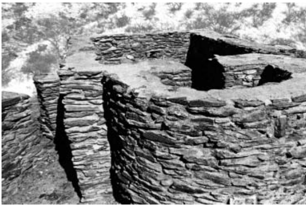
FIGURE 17. The Eros Fort outside Windhoek, built in 1893, present condition. Photograph courtesy of Dr Andreas Vogt, Windhoek/Namibia.
