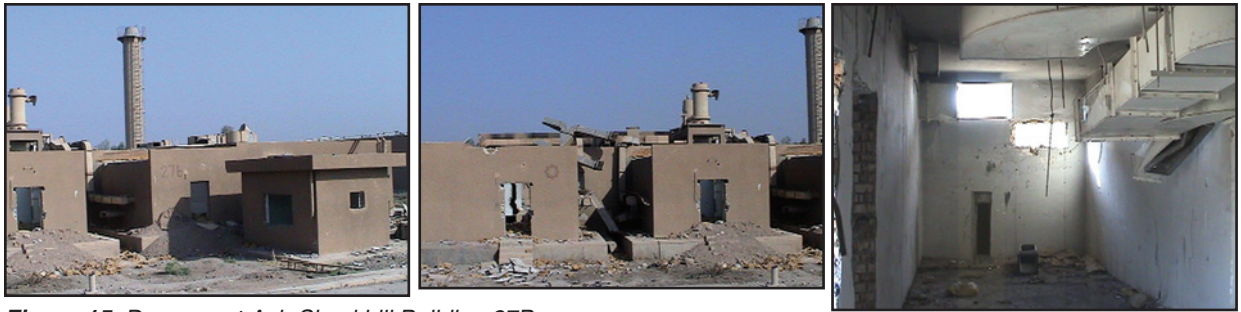
Figure 15. Damage at Ash Shaykhili Building 27B and remaining air ducting in July 2003.
