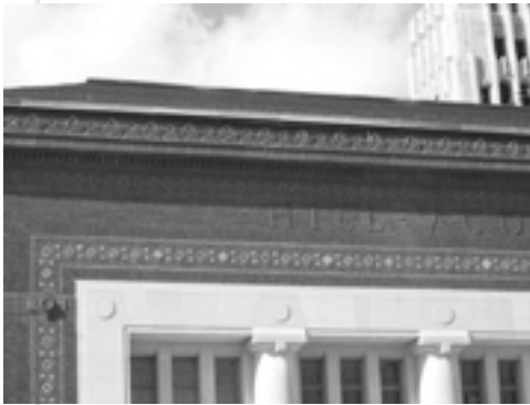
Brickwork, Hill Auditorium
