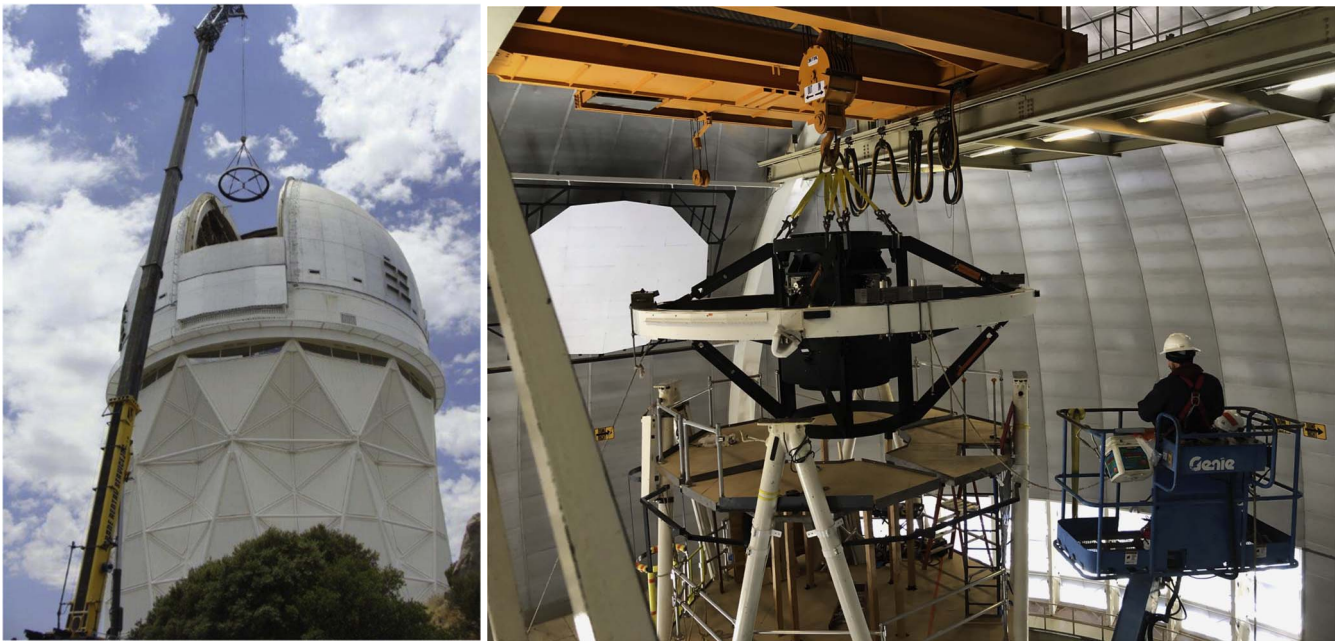
Figure 24. Installation phases of the new top ring. (Left) Transfer of the new top ring from the ground level to the dome floor via the dome slit with a 450 ton crane on 2018 June 14. The same crane was used to remove the old top end. (Right) Installation of the fully assembled, new top end with cage, hexapod, and corrector barrel to the Mayall's Serrurier truss on 2018 November 28.
