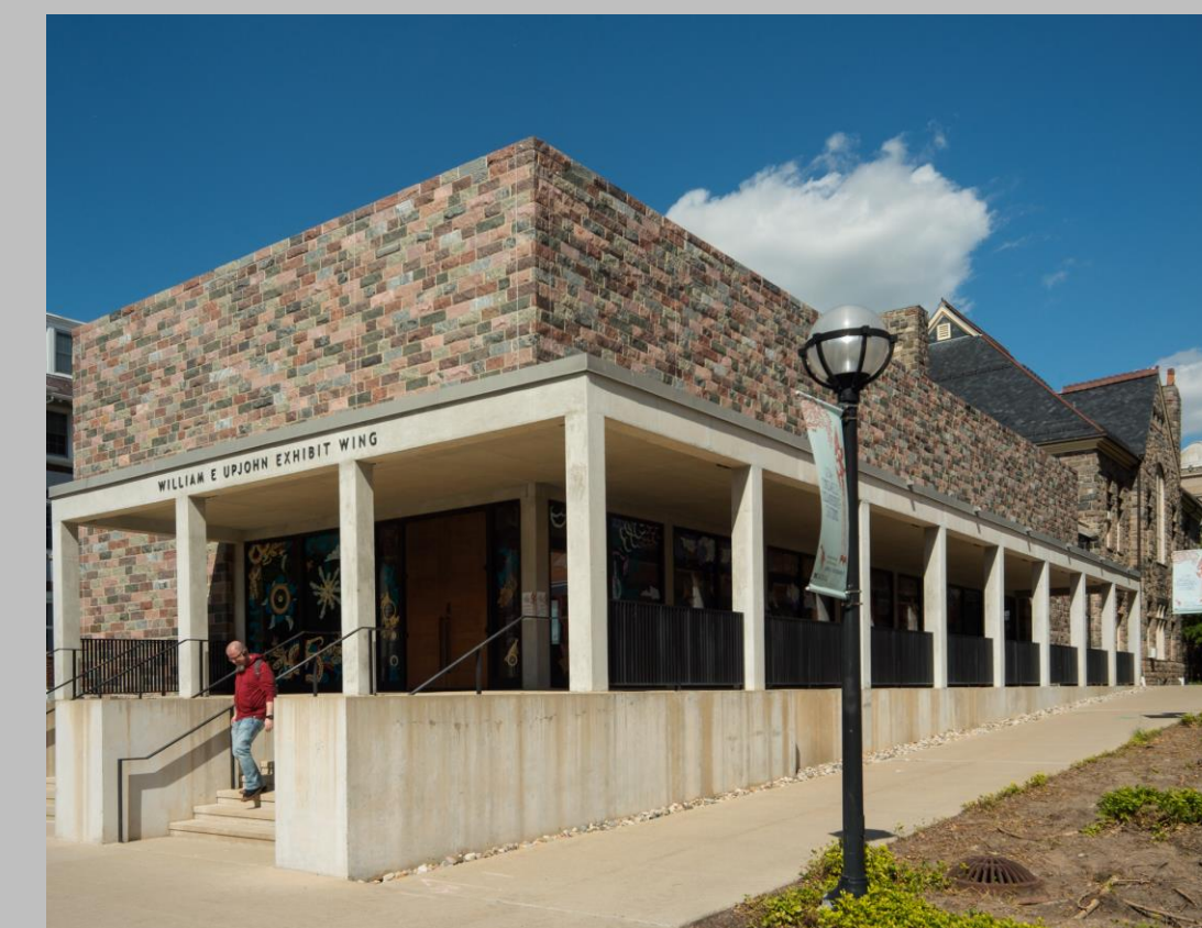
Upjohn Wing (Maynard Street entrance) Photo by Randal Stegmeyer
