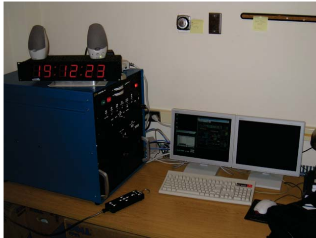
Figure 19: Telescope Control System showing the TCS cabinet and the TCS console.
