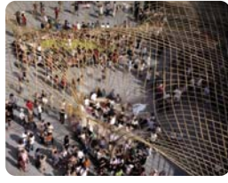
Canopy, created by nArchitects, was a temporary environment constructed of weather integrated bamboo. The bamboo structure provided shade as well as mist and fog built into the bamboo.
