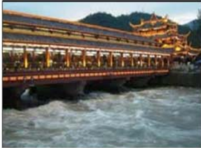
Fig.3 : Dujiangyan Dam in China
