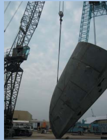
An overhead gantry crane and a crawler crane are used to flip the bow section.
