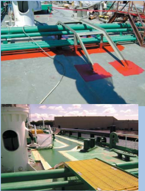
Figure 2. This ramp, designed by intern Tera Herman, allowed for a method to move materials over a series of pipes.
