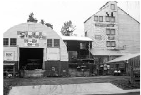
Figure 29: Adaptive reuse of an old railroad grain elevator into a mixed use garden store and residence: Stookey's Feed and Garden, Moscow, Idaho
