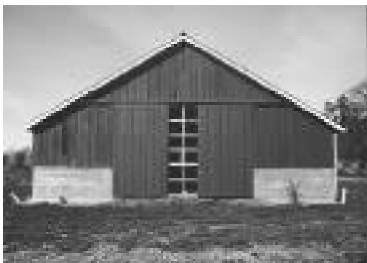
Figure 38: South elevation of stall barn
