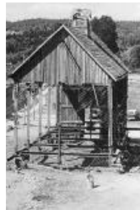
Figure 36: Stabilizing the loft barn (KPG, Inc.)
